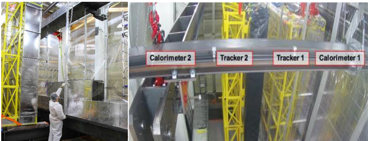
Figure 3: Left: a view of the installation procedure of Optical Modules in the calorimeter wall. Right: Side view of the two calorimeter walls and the two tracking chambers already installed at Modane.
