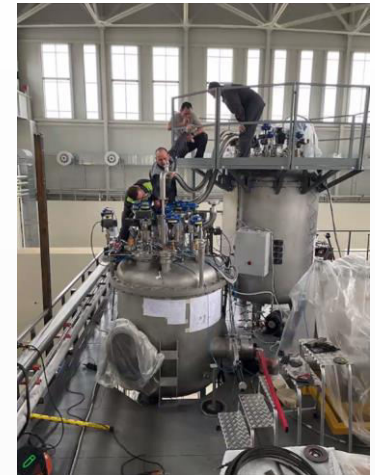
Cryogenic platform with Satellite Refrigerator and Control Dewar
