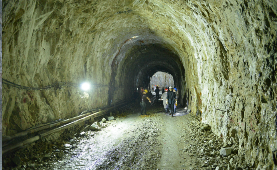
Access tunnel to the experimental hall
