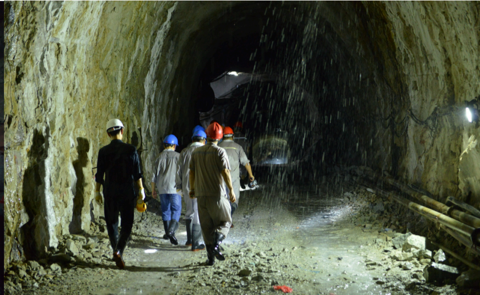
One of the service tunnels
