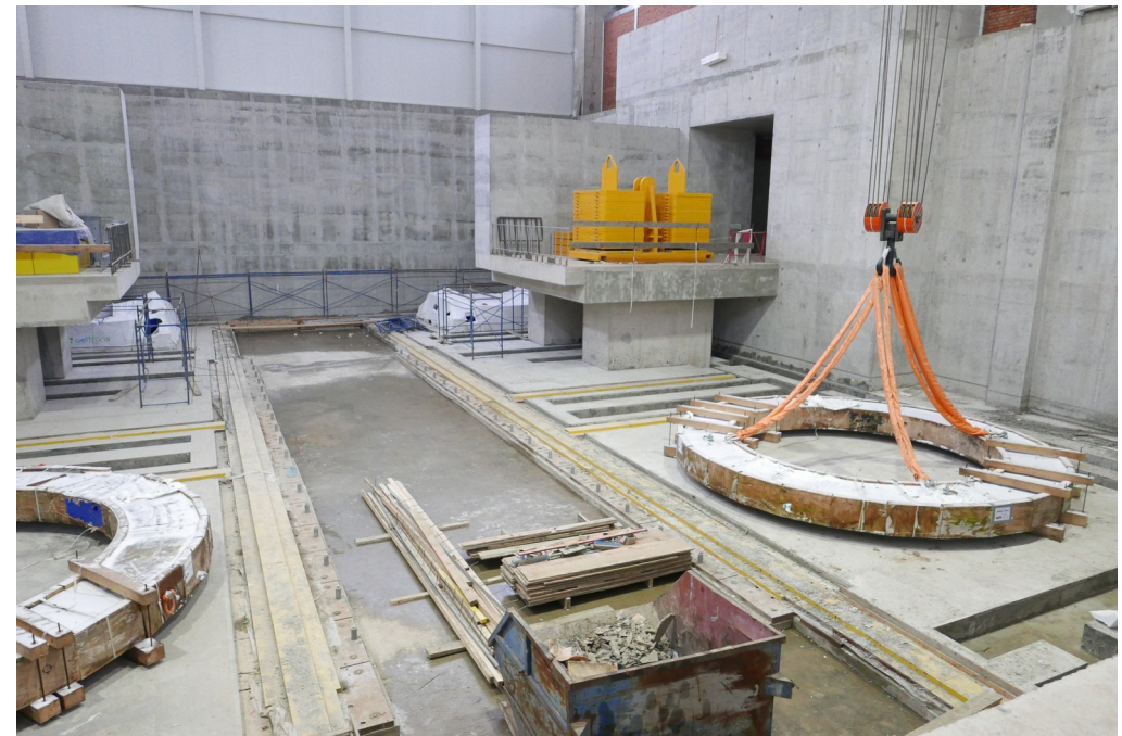
Transportation of MPD Magnet Yoke parts into the MPD pit (inside MPD Hall)
