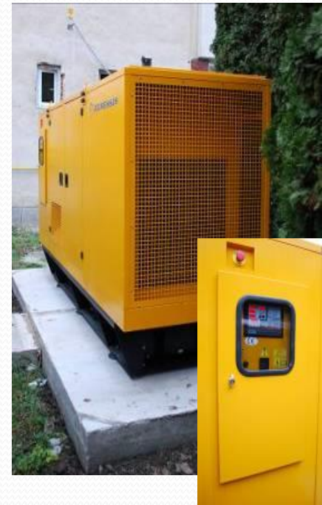
Power generator 275kW
