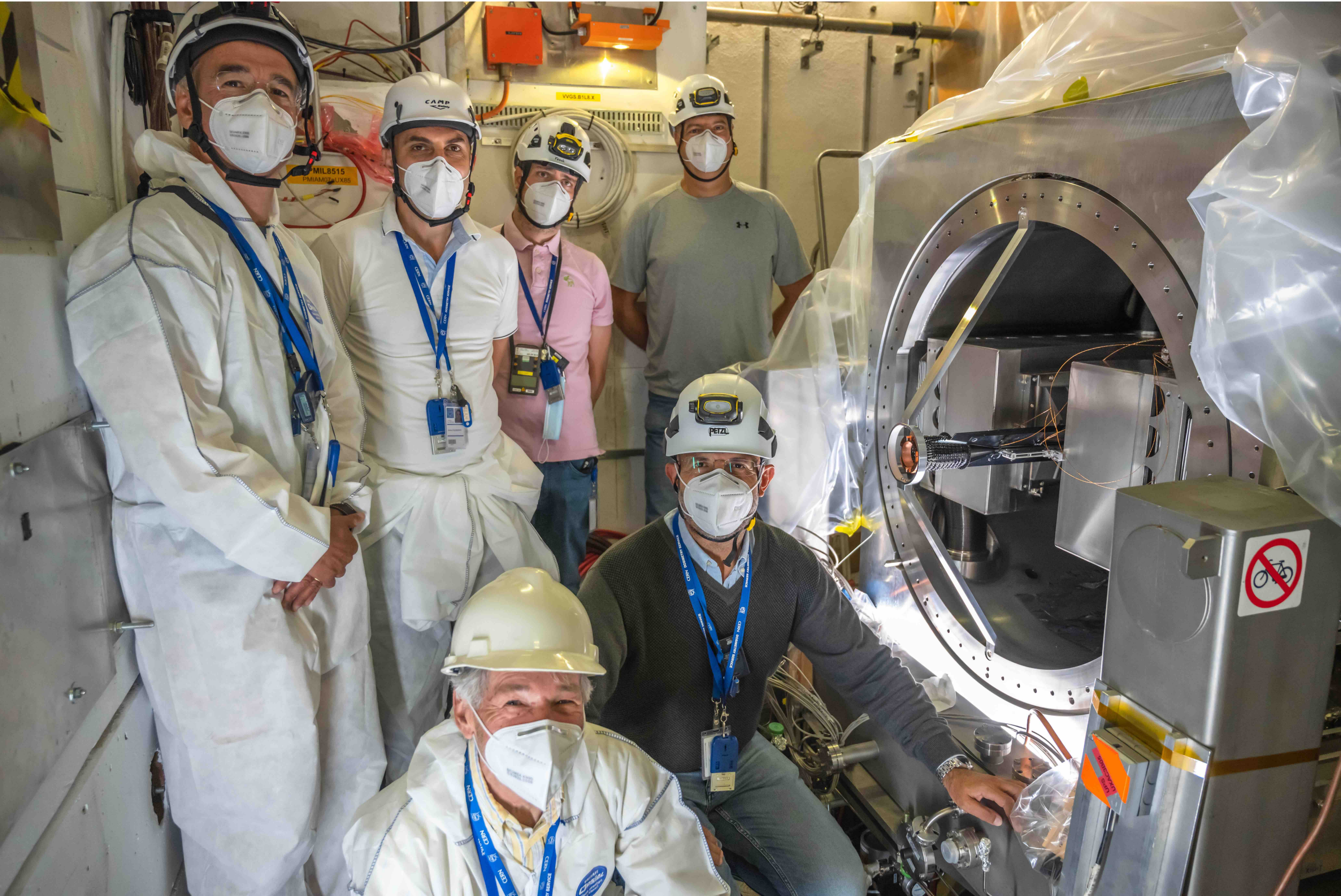
During the installation
