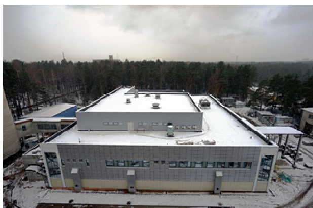
Building of the Superheavy elements factory
