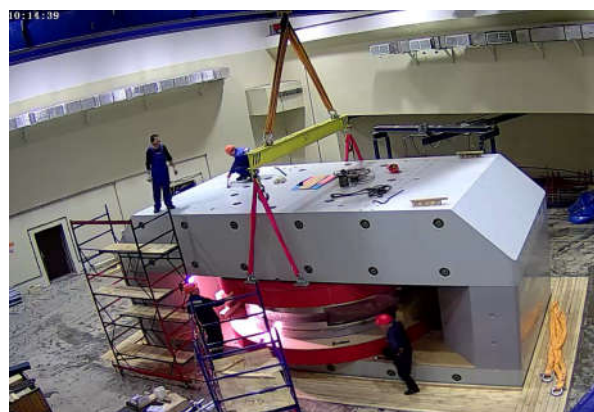
Assembling of the main magnet of DC-280 cyclotron
