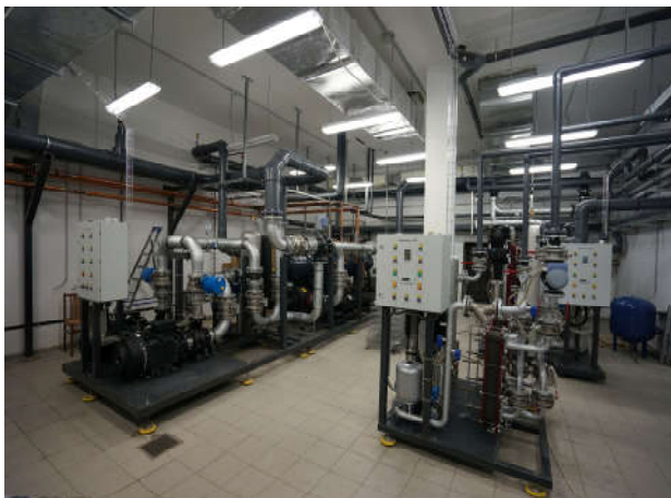
Installation of the water cooling system
