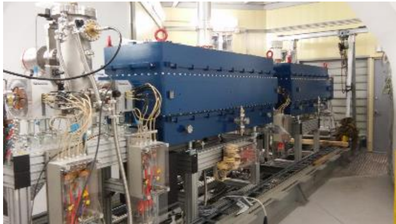
Figure 3: Heavy ion linear accelerator of the NICA collider complex
