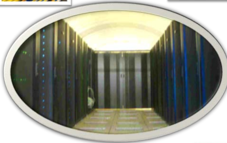
High Density Heat Containment System
