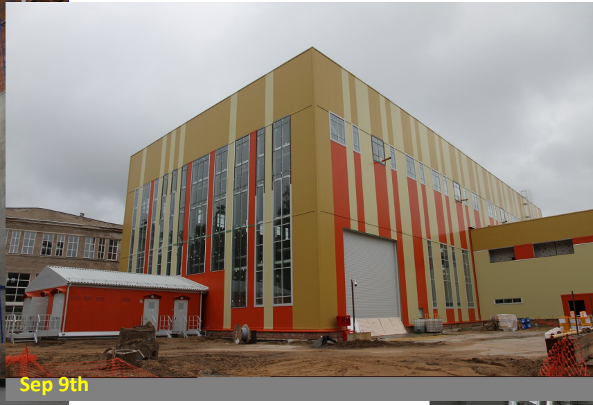
Exterior of the MPD Hall Building and high voltage connection housing
