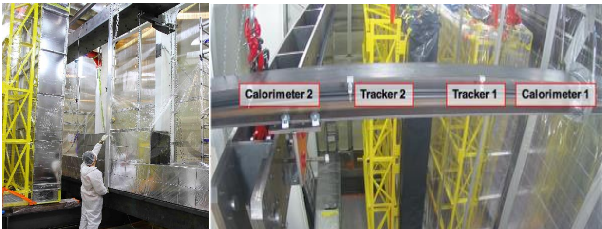
Figure 3: Left: a view of the installation procedure of Optical Modules in the calorimeter wall. Right: Side view of the two calorimeter walls and the two tracking chambers already installed at Modane.
