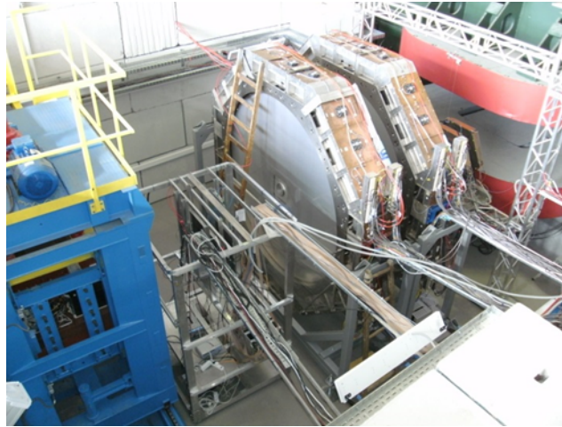
Fig. 2.2.2.37. Two DCH chambers installed in the BM@N experimental zone.
