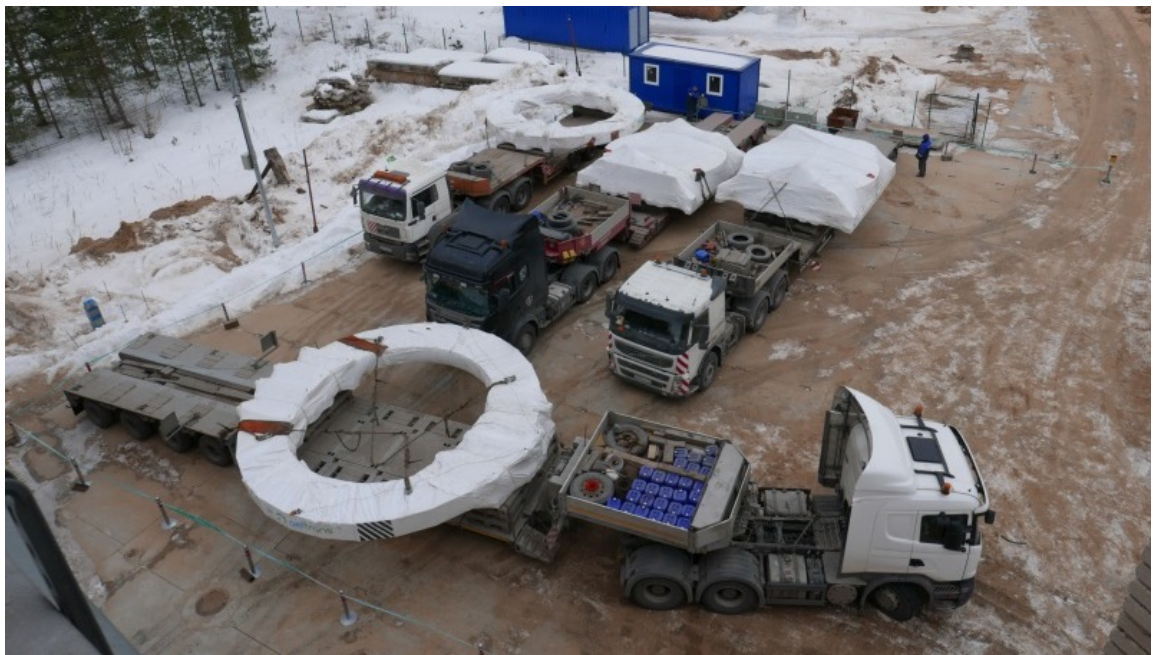
Fig. 2.2.1.16. Support rings and poles in the temporary customs control zone (March 2019).
