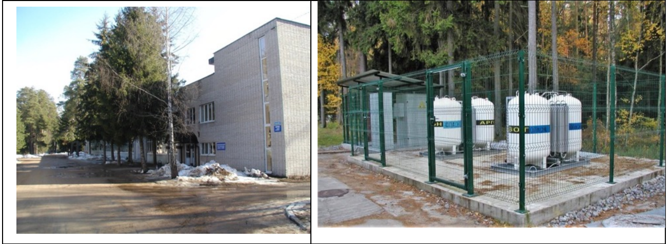
Fig. 2.2.1.28. Building 217 common view and TPC gas supply system
