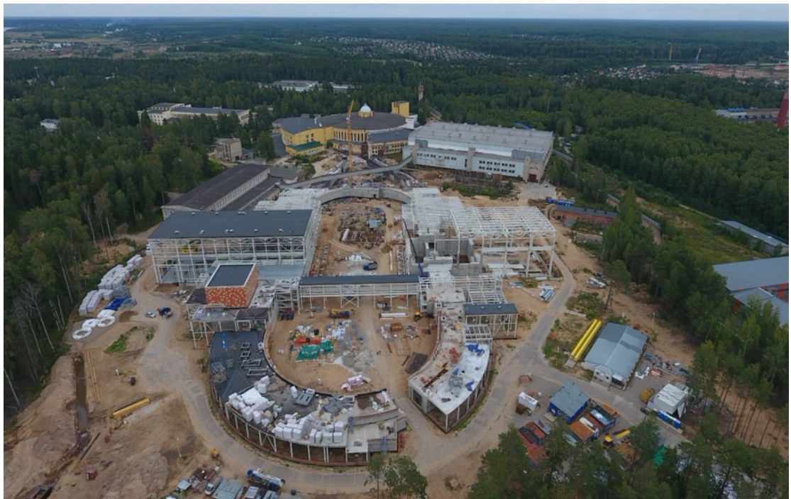
Fig. 2.3.1.1. General view of the construction site (August 2019).
