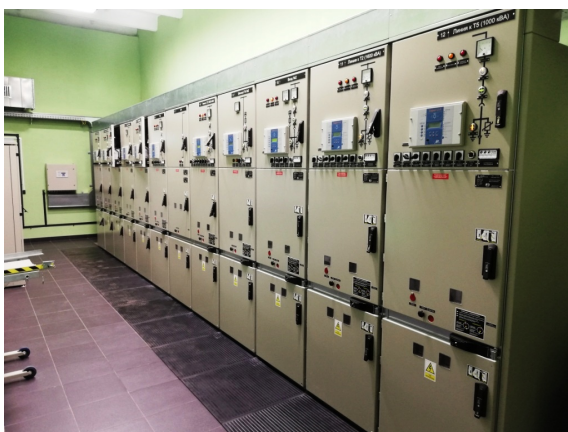
Switchgear 6kV substation "K"
