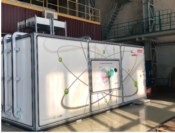
MDC outside view.
