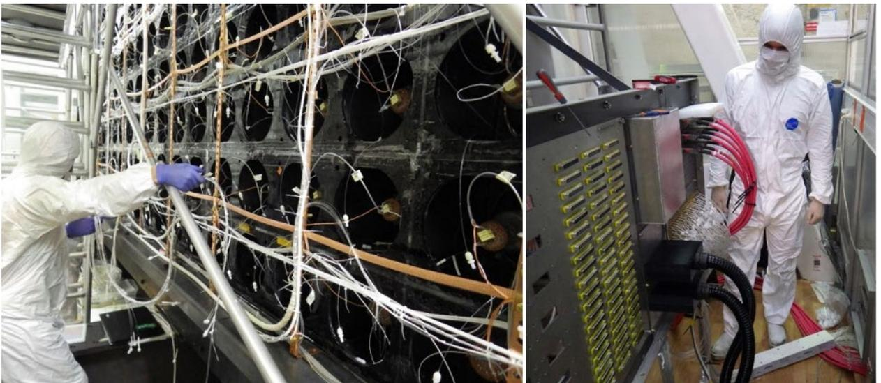
**Figure 8.** Installation of fibers (left) and light injection system (right).
