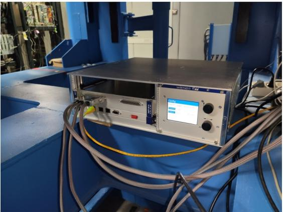
New WIENER MPOD power supply unit has been installed
