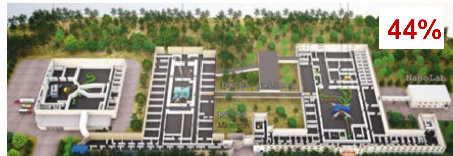
Full-scale realization of the DRIBs-III project
