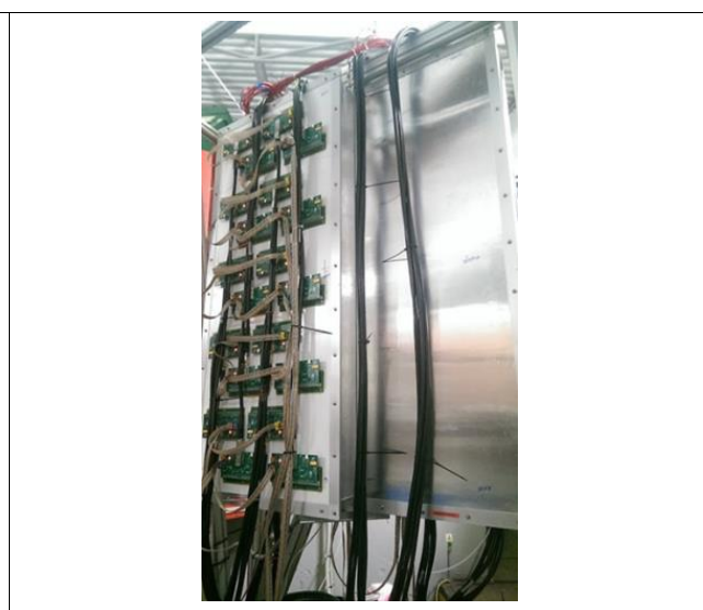
Fig. 3.5.2b Real view of a half part of the TOF400 system
