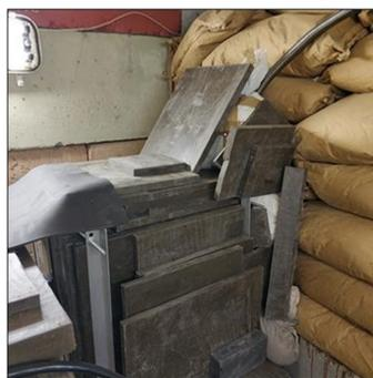
**Fig. 1.** The neutron protection is installed near the local beam shutter inside the experimental room of the 11b channel.
