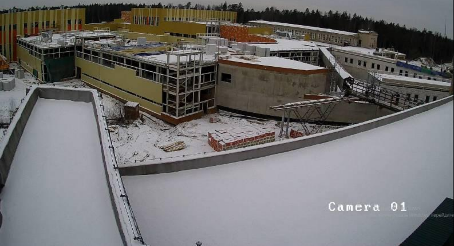
General view of the collider construction site in December last year.
