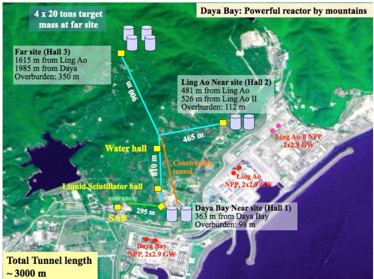
Fig.2.3.1 Reactor complexes Daya Bay, Ling Ao and Ling-Ao-II. Antineutrino detectors of Daya Bay experiment are located in three experimental halls: two near and one far. Two near halls contain a pair of antineutrino detectors each. The far hall contains four antineutrino detectors. The far hall is shielded by 350 m of rock from cosmics.
