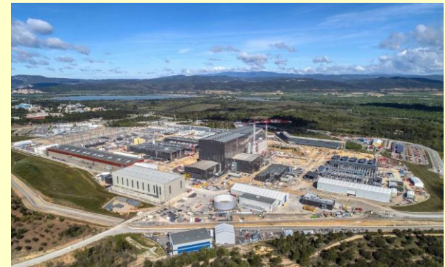
ITER construction side
