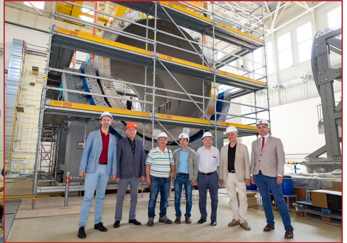
Installation of the MPD Superconducting coil inside the iron Magnet Yoke in MPD Pit 29 July 2021
