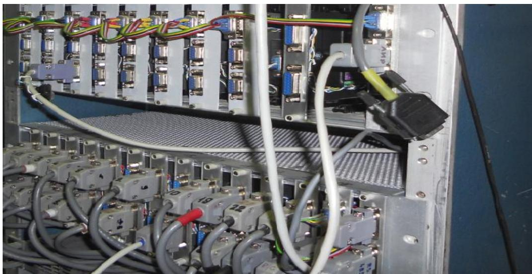
**Fig. 6.1.** Control system of actuators of the REMUR spectrometer for 32 control channels.
