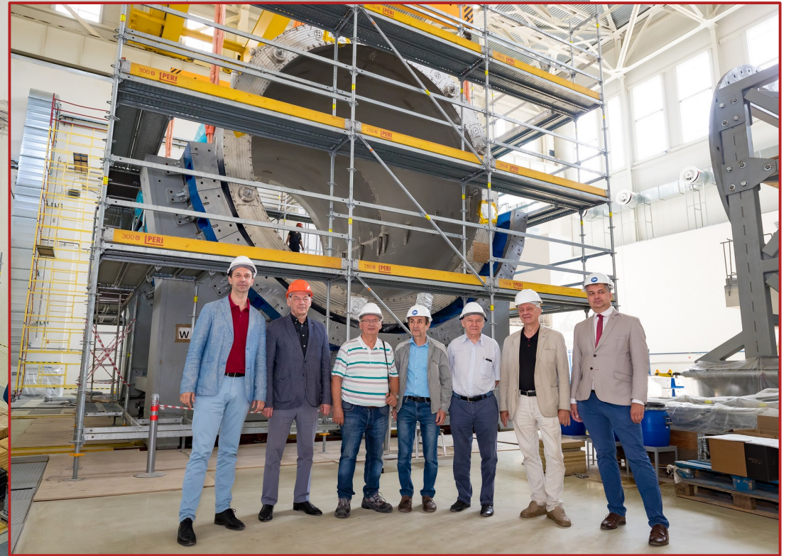
Installation of the MPD Superconducting coil inside the iron Magnet Yoke in MPD Pit 29 July 2021
