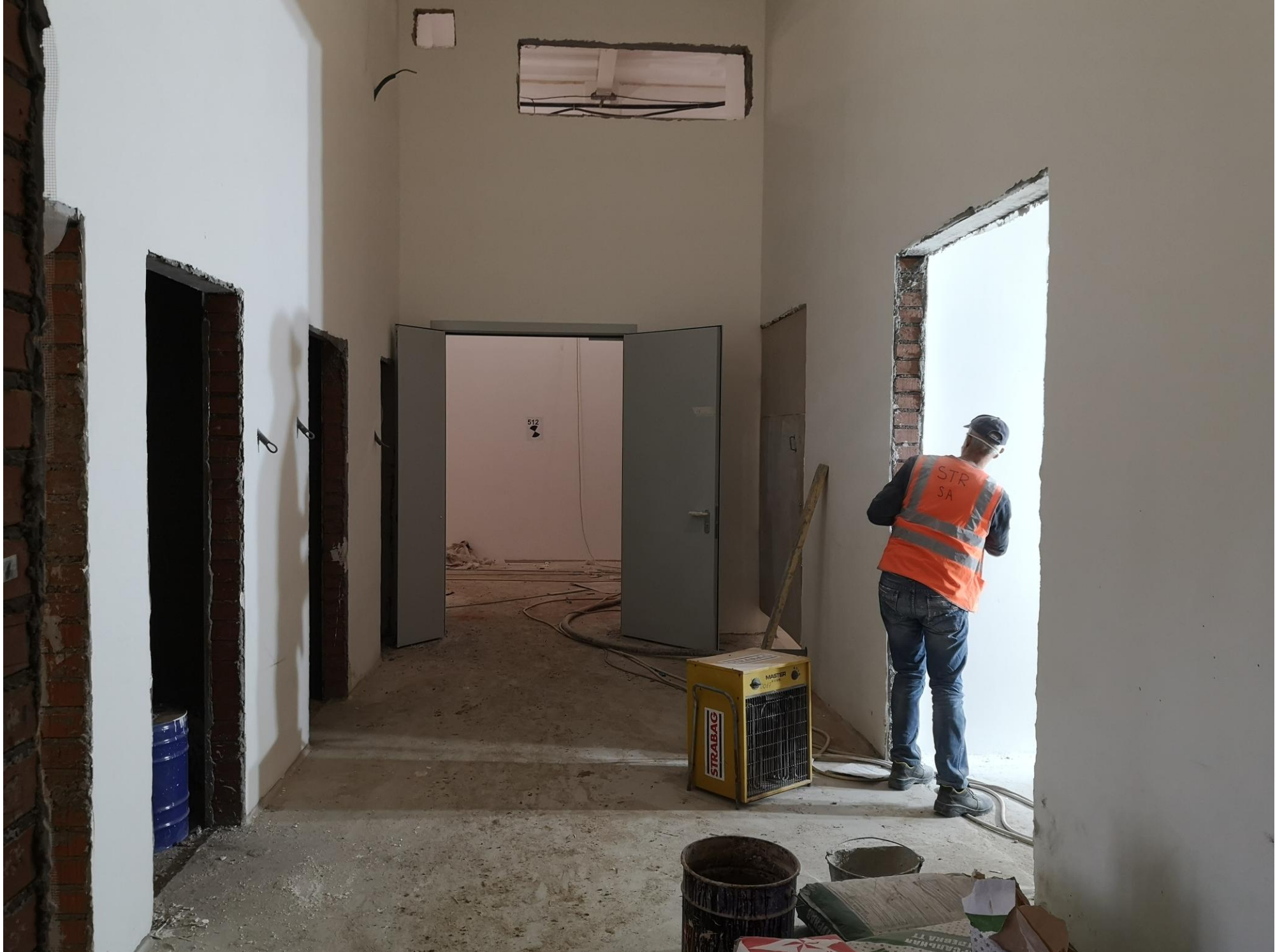
Interior decoration of the control room: 19.11.2021
