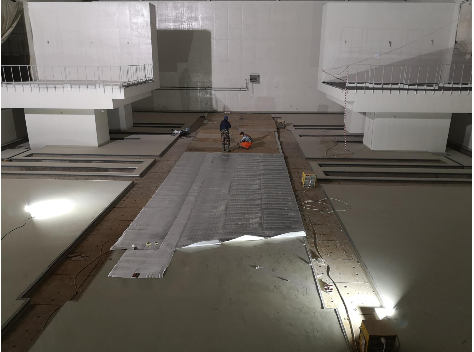
We have provided protection for the floor from mechanical damage. December 2021.
