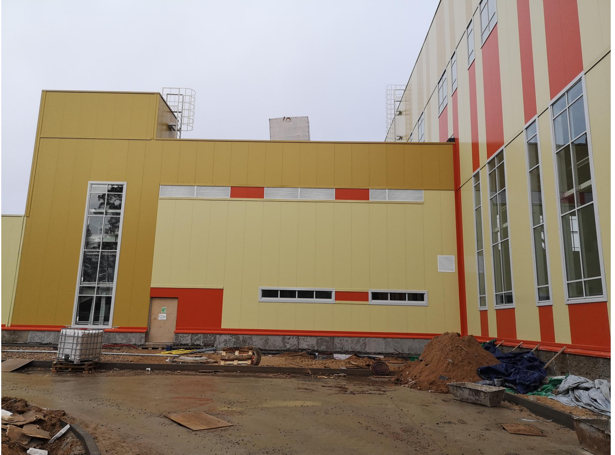
Main entrance in Control Room
