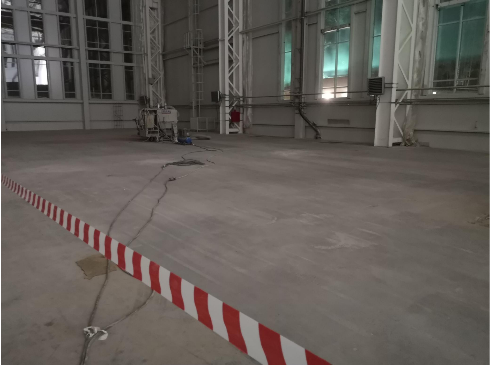
Grinding the floor in the main hall. 08.12.2021 (a week ago).
