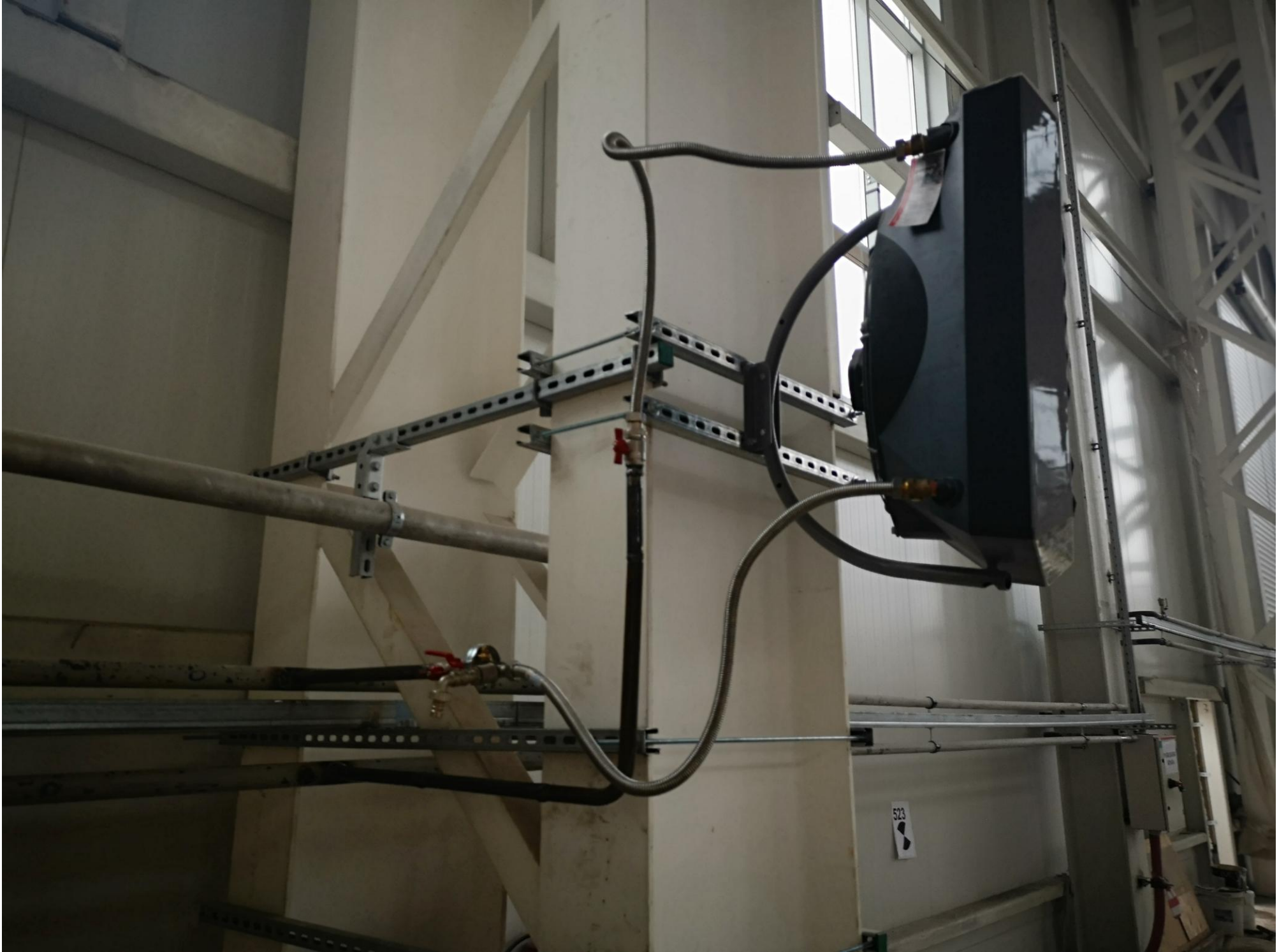
Water-type heating convectors are in the process of being connected
