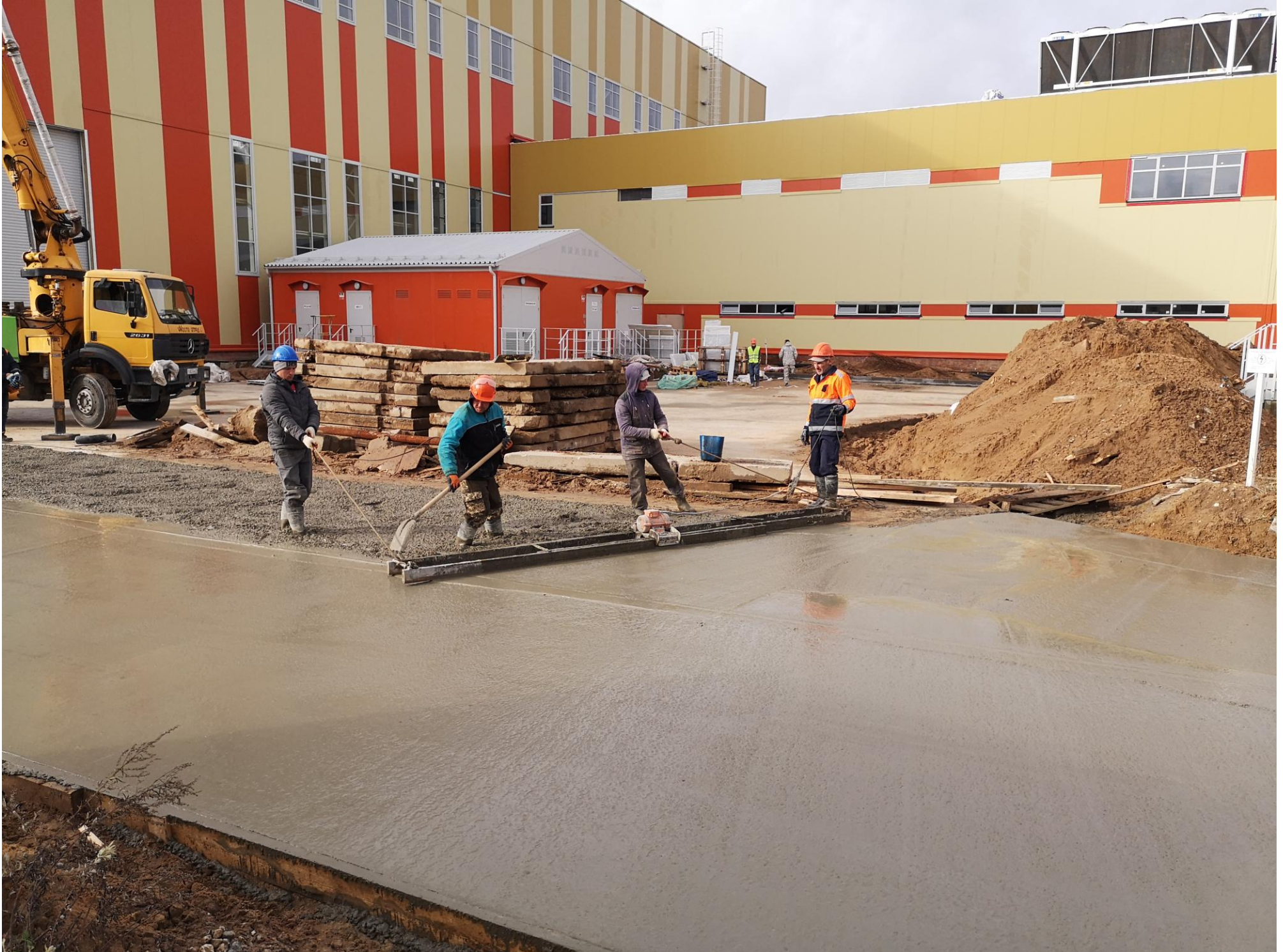
Access roads to the building are poured with concrete: September 2021
