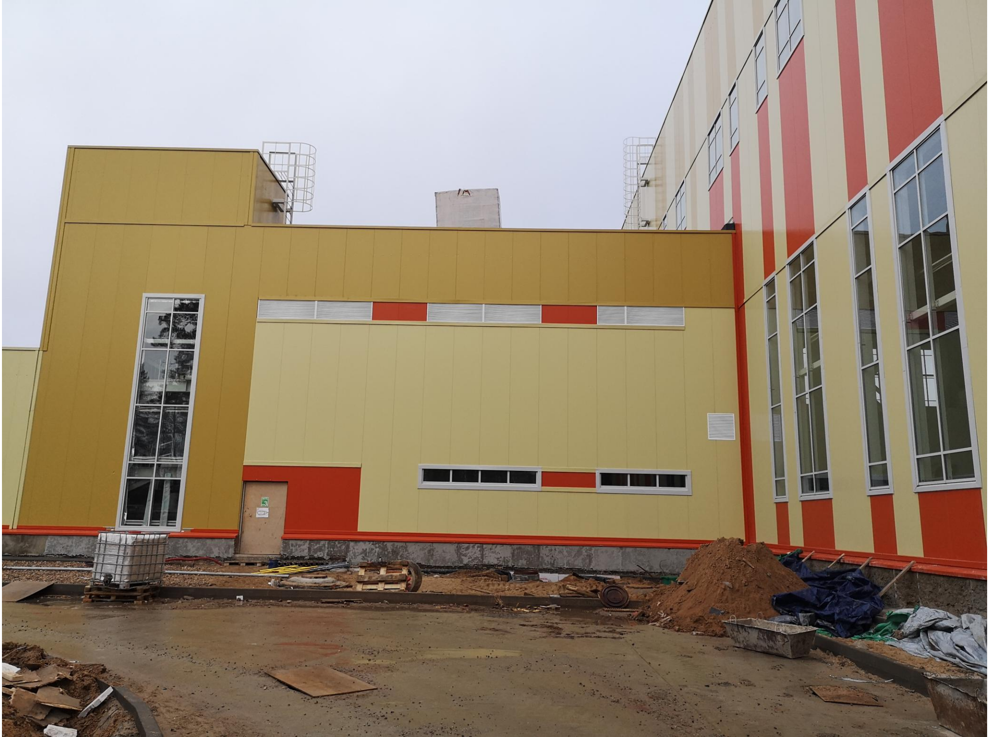
Main entrance in Control Room
