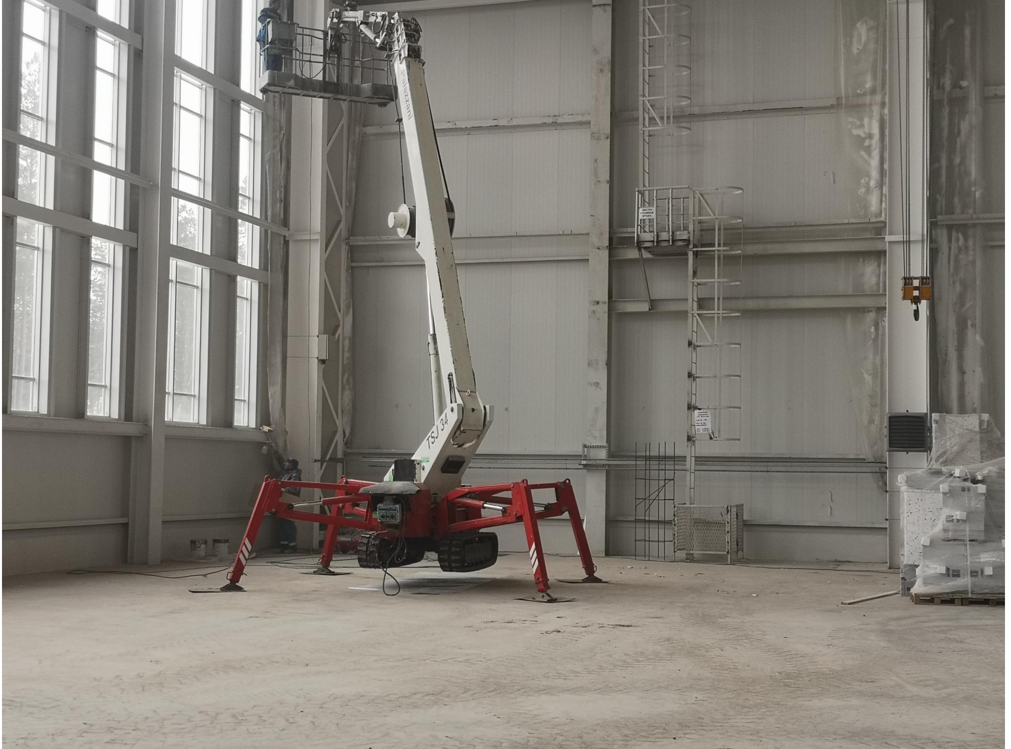
The interior painting of the walls of the hall is being completed.
