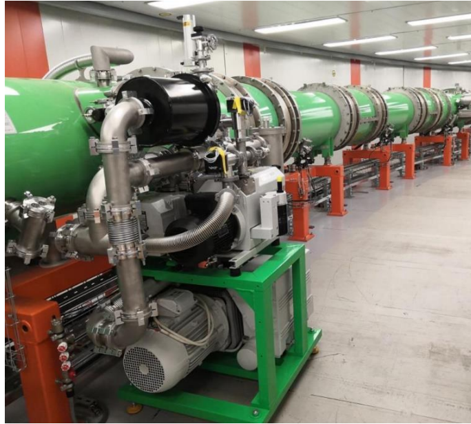
Fig. 3. The Booster cryo-magnetic system in assembly
