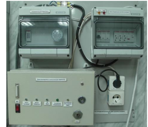
Interlocking and alarm system switchboard
