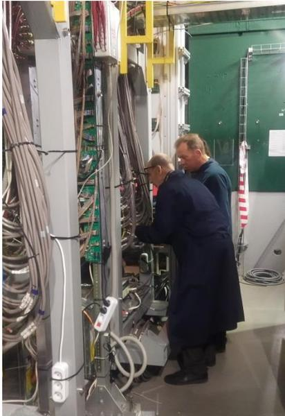
Researchers are connecting and testing the DCH after rearranging and aligning the detectors
