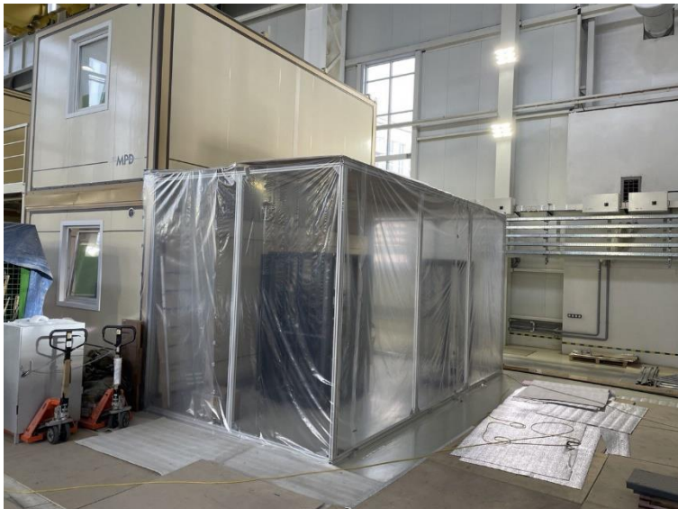
"Tent" for assembling gas system in the MPD hall
