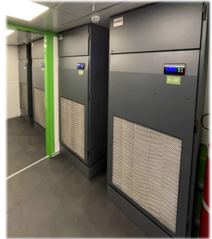
Quad Precision Air Conditioners N+1 redundancy
