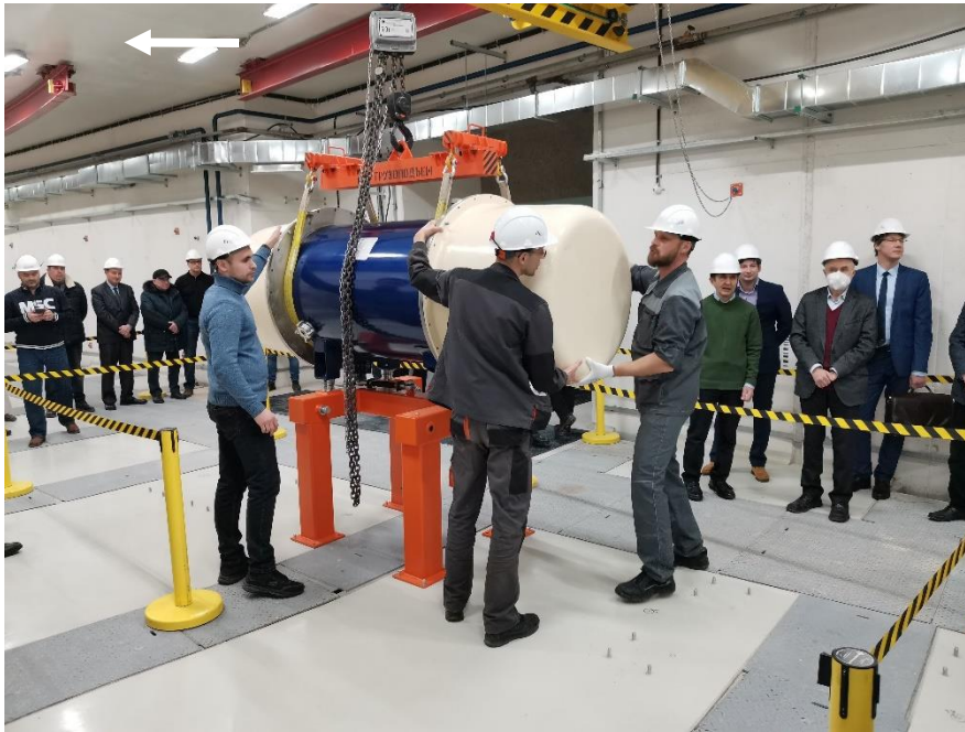
Fig. 8. 28 December, 2021. Installation of the first collider dipole magnet in the tunnel
