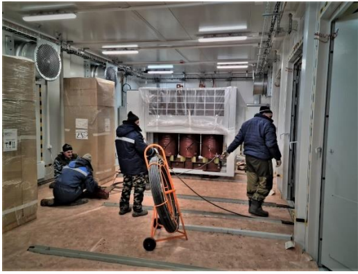
c) installation of transformers
