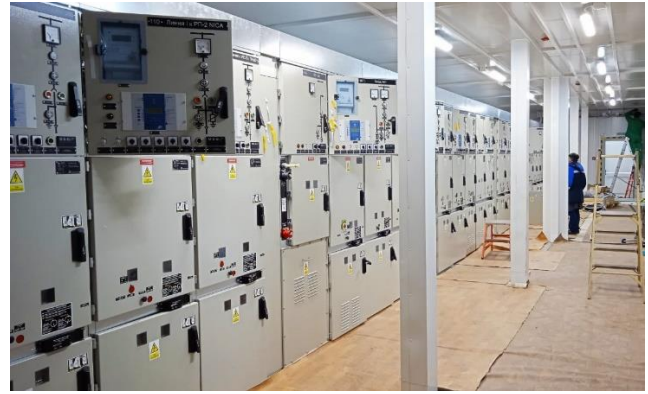
d) installation of PS15 cells
