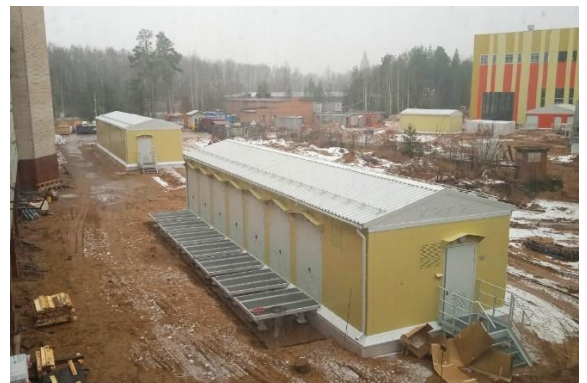
b) Transformer and PS15 buildings
