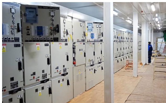
Fig. 7. Installation of the power supply units.
