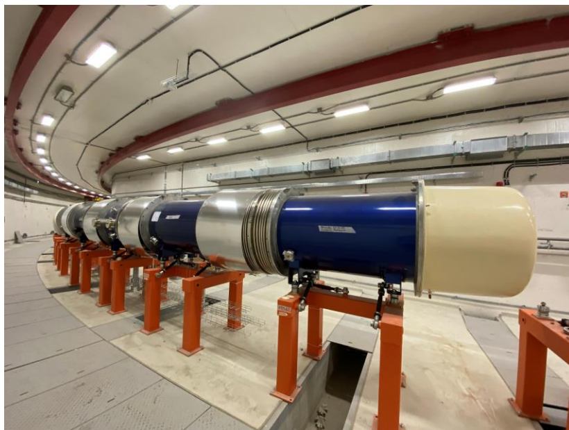
Fig.13. The collider arc dipole magnets in the tunnel.
