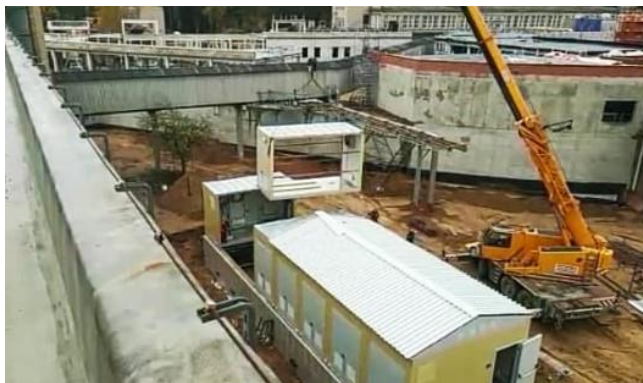
a) installation of Transformer building
