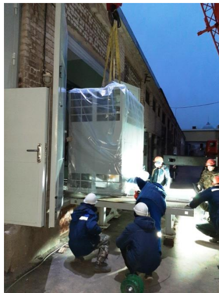
Fig. 17. 15.11.2022: Installation of the 1.6 MVA transformer in the chamber of building 1A.
