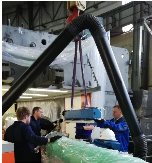
Fig. 2. Installation of the septum magnet of the fast extraction system
