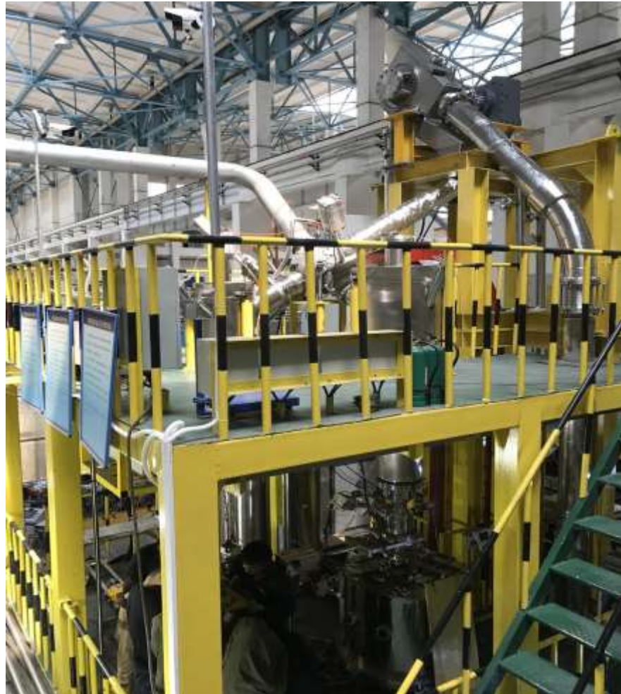
(Pipe Chain Lift)
