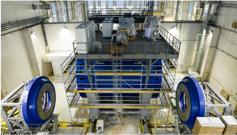
Top platform (cryogenics, power supplies, control system)
