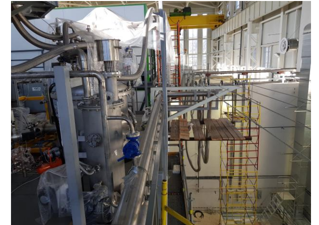
Strings for cryogenic pipes and cables hold
