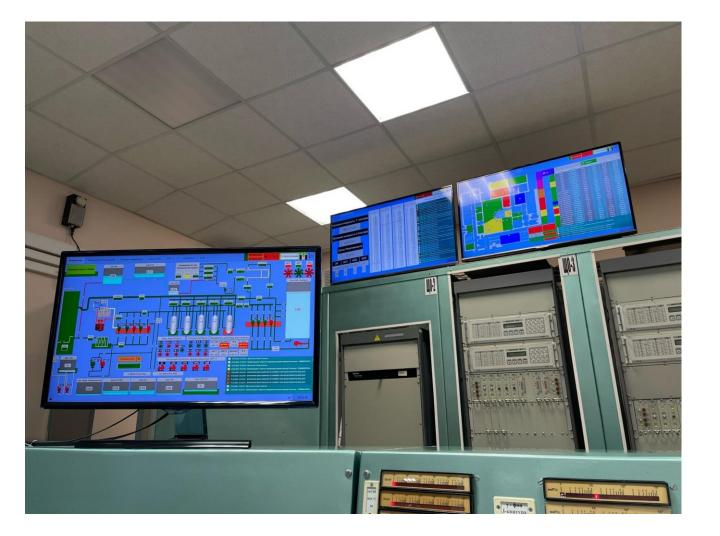
Simple SCADA software complex was developed in 2019 by service department of IRT-T for simplification of management and informational support for the personnel who is responsible for reactor operation.
