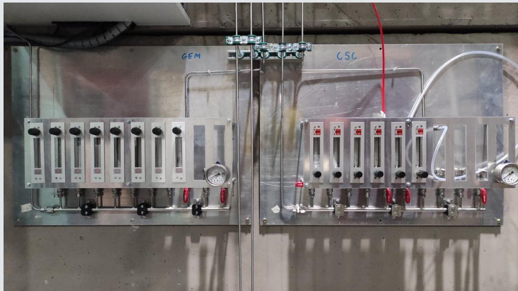
Gas collectors: GEM – left, CSC – right
