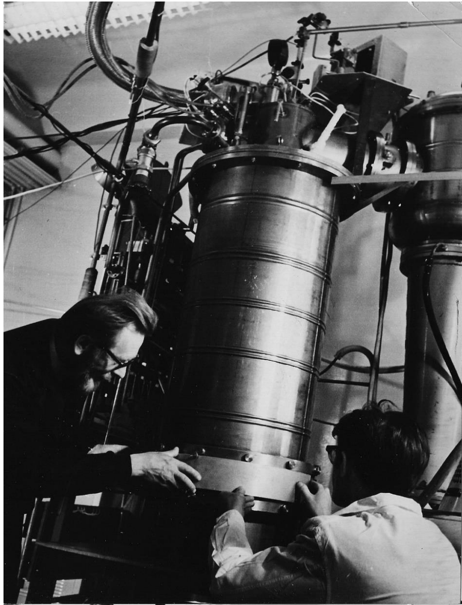
The first Frozen Polarized Target (1975) during tests preparation (B. Neganov and N. Borisov)
