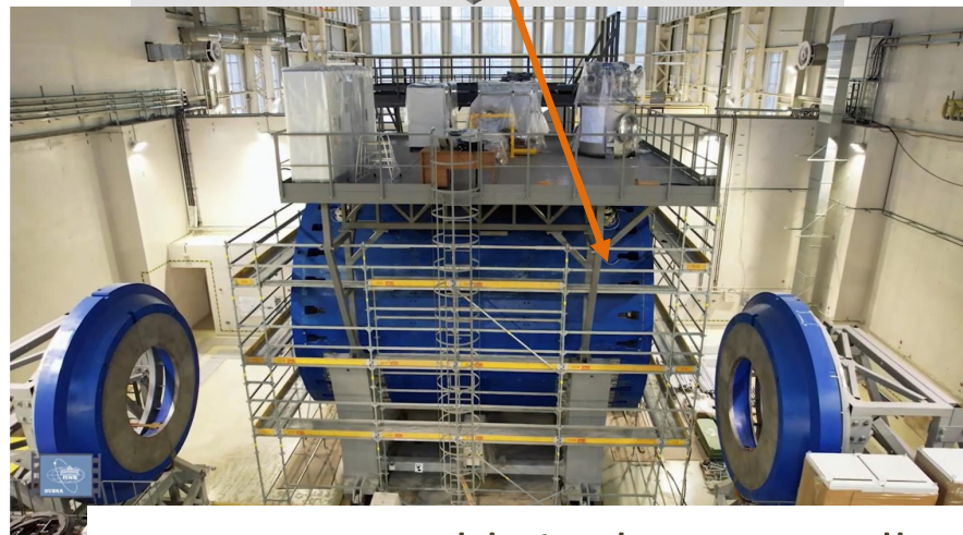
Magnet assembly in the MPD Hall
