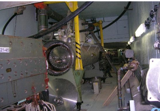
RF deflector in the beamline
