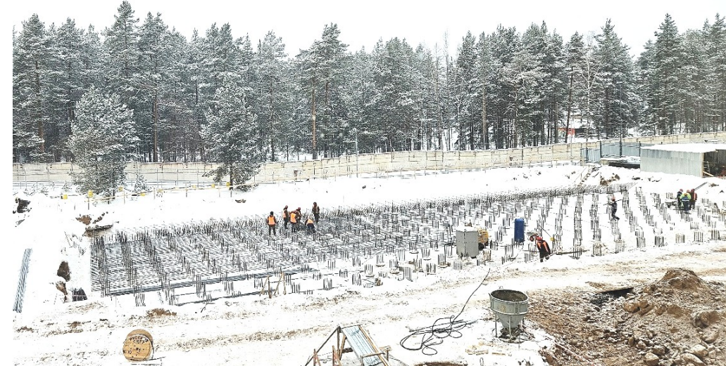
Completion of the pile field 08.12.23
