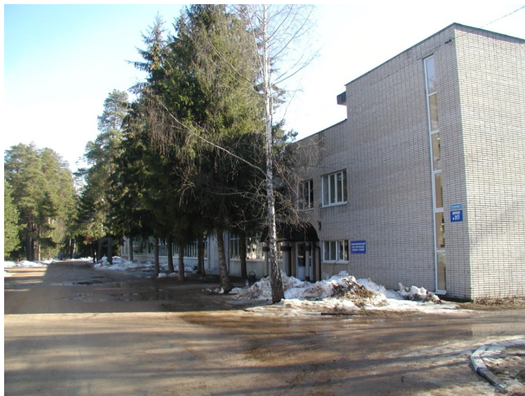
Figure 13.1: Building 217 common view
