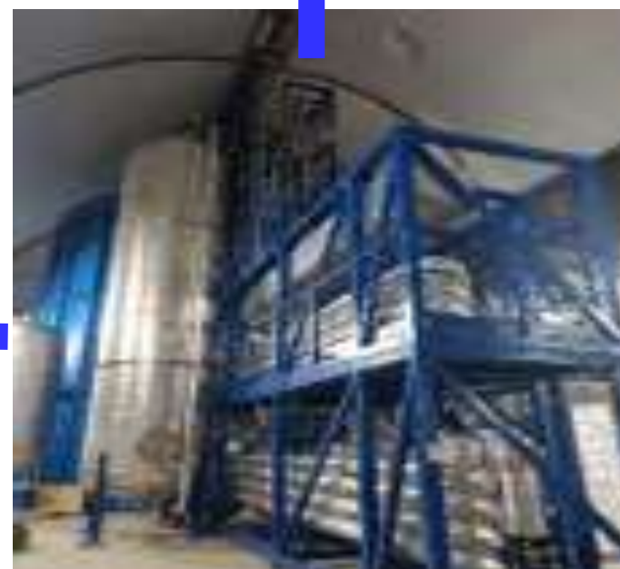
4) Gas stripping to remove Rn and O 2
