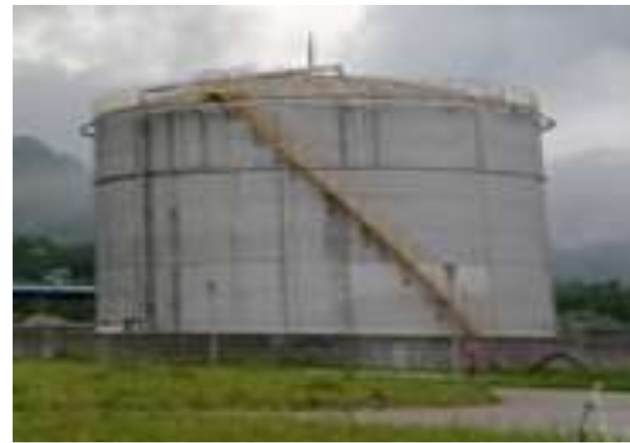
5000 m 3 LAB storage tank
