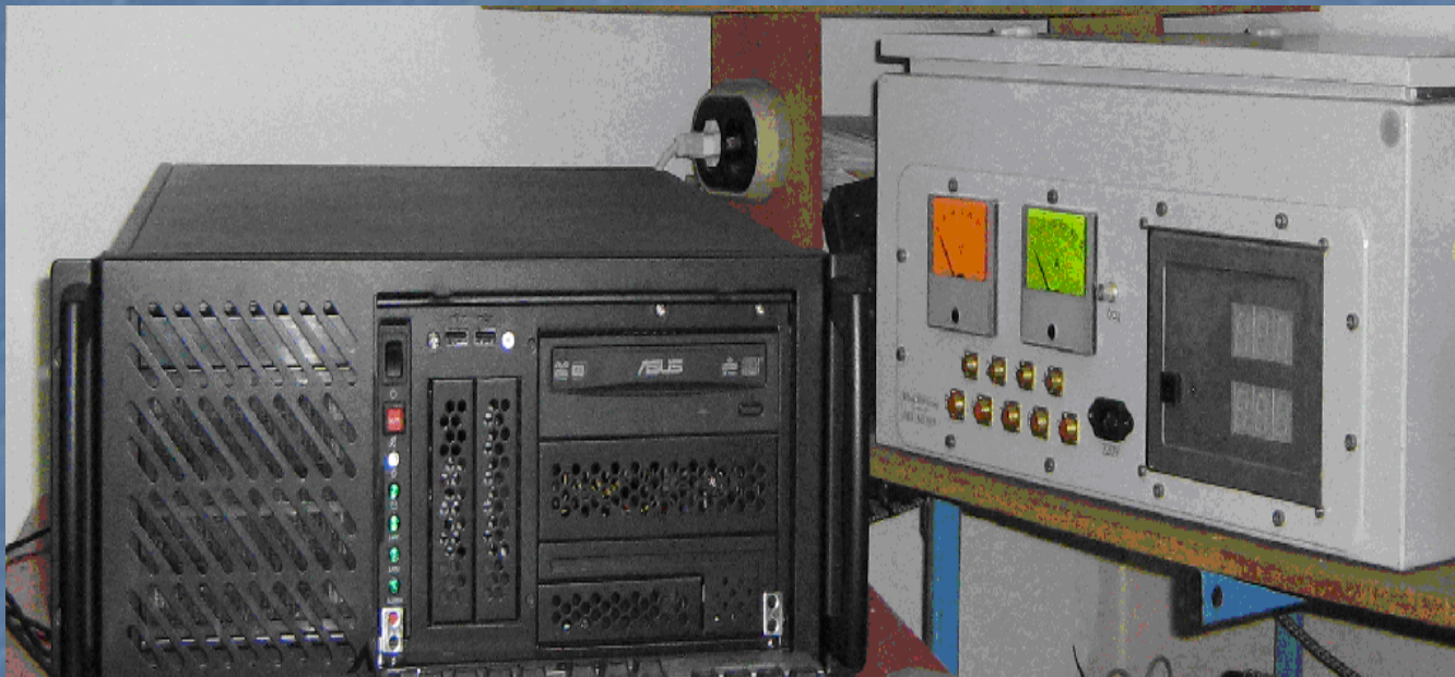
Fig.1 500 Amper generator with Industrial PC
