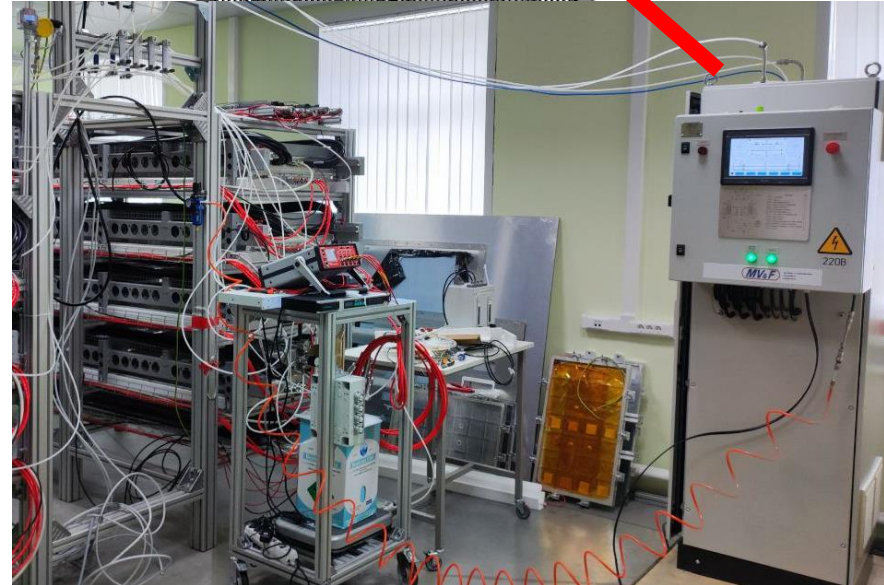
Rack #4 – Gas mixture purifier
