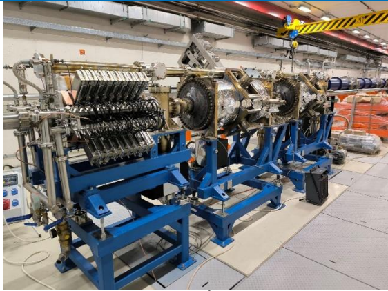
RF1 and RF2 in tunnel
