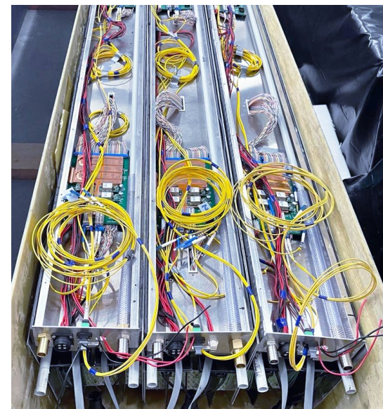
ADCs & cooling system
