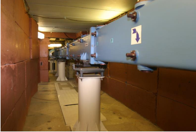
Curved mirror neutron guide
