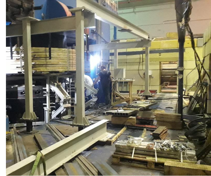
Upper coil lift process
