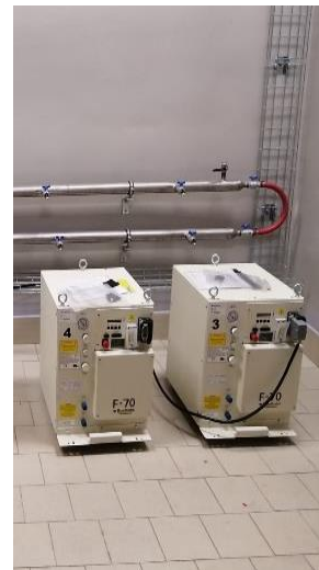
Cryopump compressors
