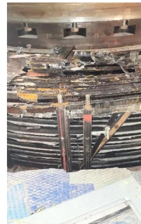
Dismantling of old main magnet coils
