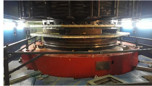
Dismantling of vacuum chamber
