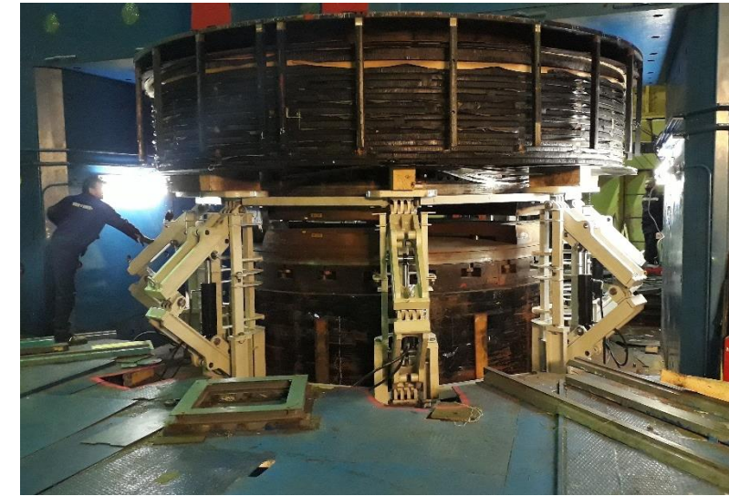
Descent of the coil by lift system
