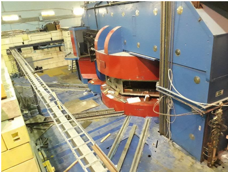
View after dismantling of RF resonators
