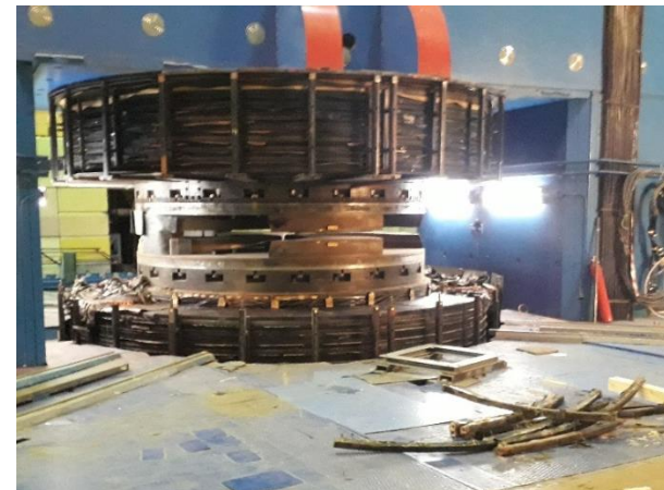
Dismantling of old main magnet coils
