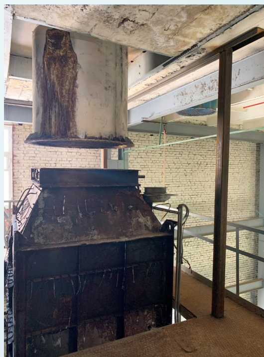
Preparing the air heat exchanger for dismantling.
