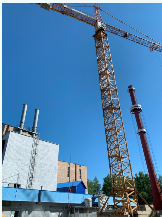
Tower crane near the reactor.
