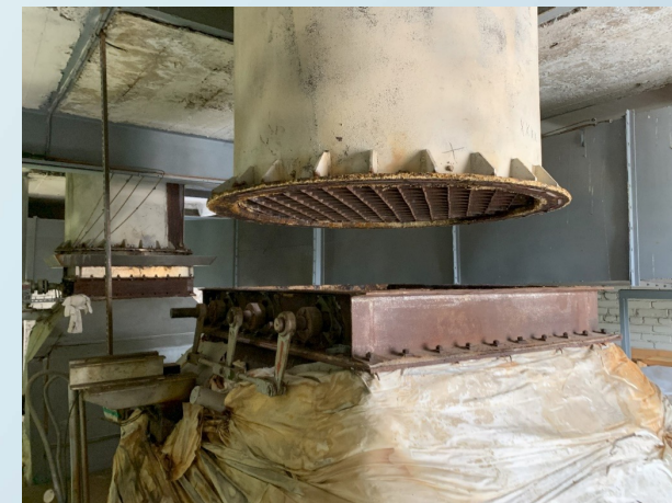
Removing the insulation of air heat exchanger.
