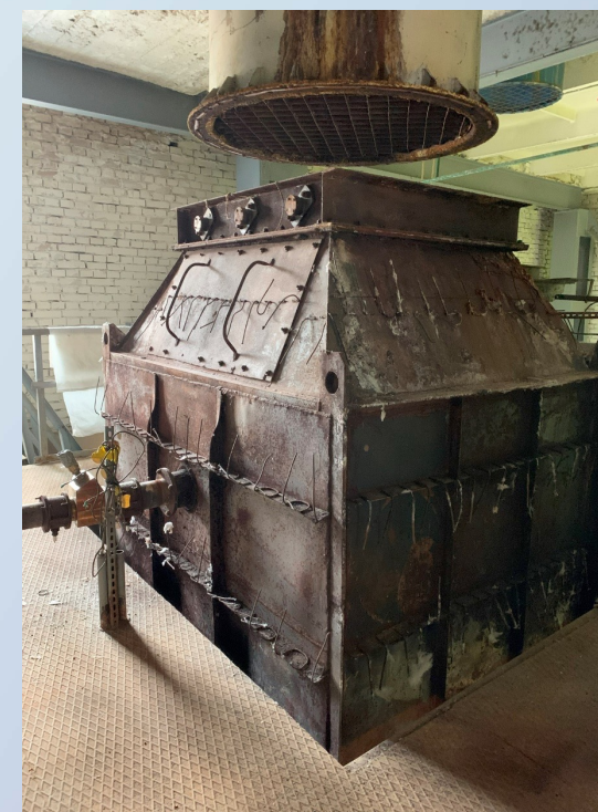
Preparing the air heat exchanger for dismantling.
