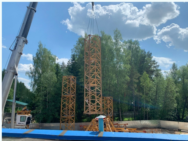
Assembling of a tower crane on-site.
