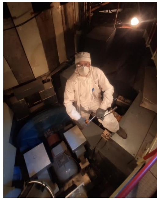
Pic. 3, 4. Replacing the grease of the bearings of the background HRFD chopper.
