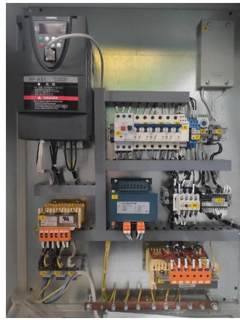
Pic. 2. The Toshiba Tosvert VF-AS1 frequency converter.
